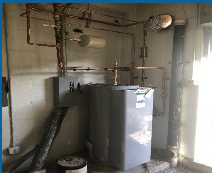
Water Heater Installation
