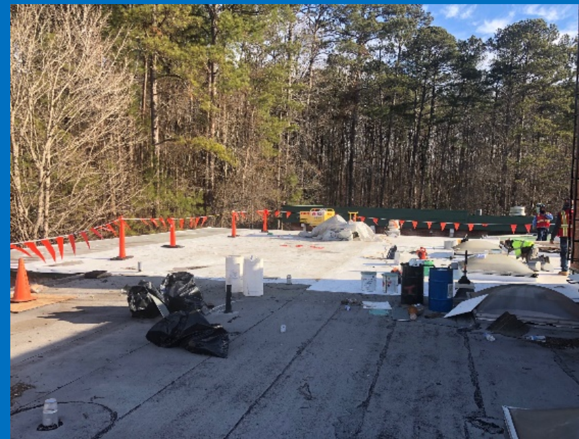
TPO Roofing Replacement
