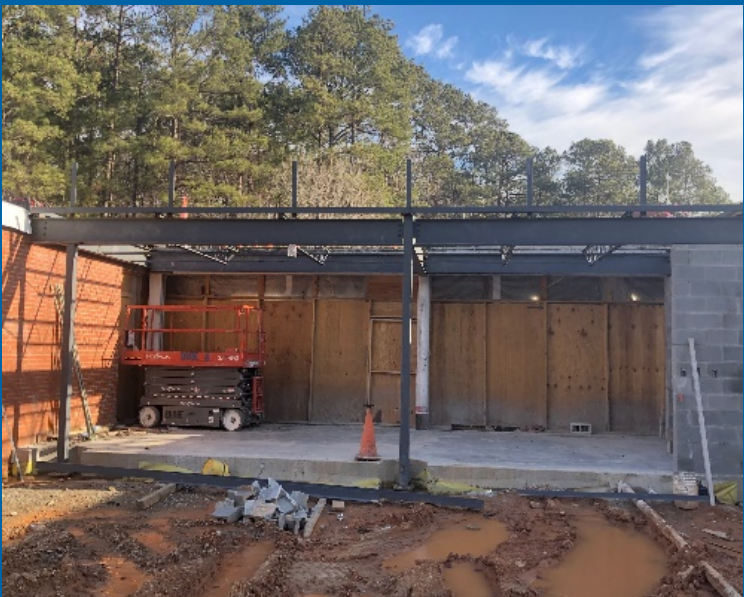
Main Entry Steel Addition
